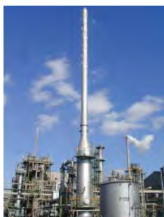
Pollution prevention investment Catalytic combustion facility for detoxification of gas emitted from production processes
