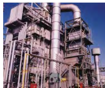
Mizushima Plant Exhaust gas denitrification unit
